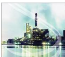
Building & Industrial Plants
